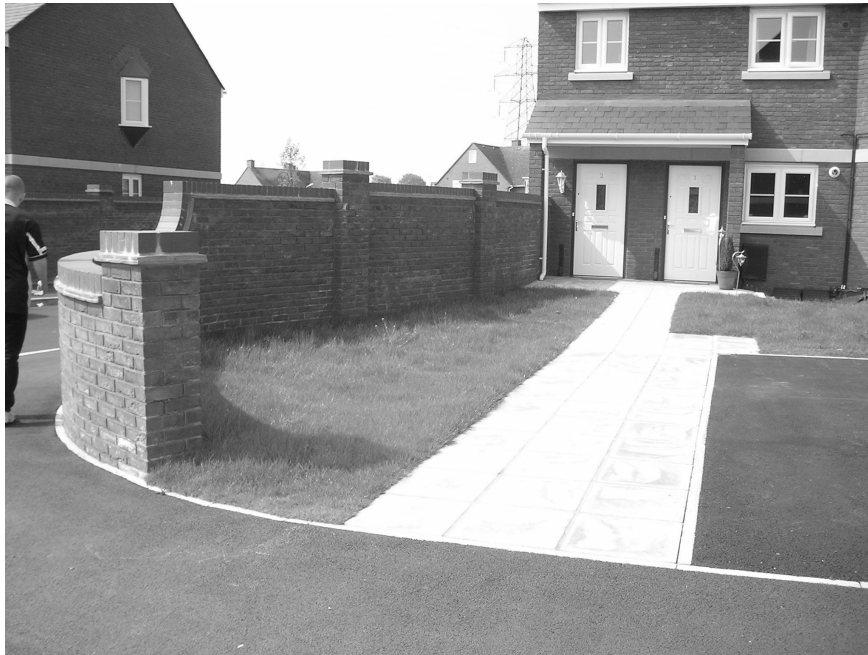
Seabrook Mews, Topsham Road
